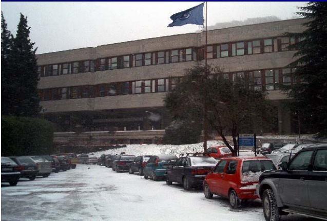
ICTP Main Building
